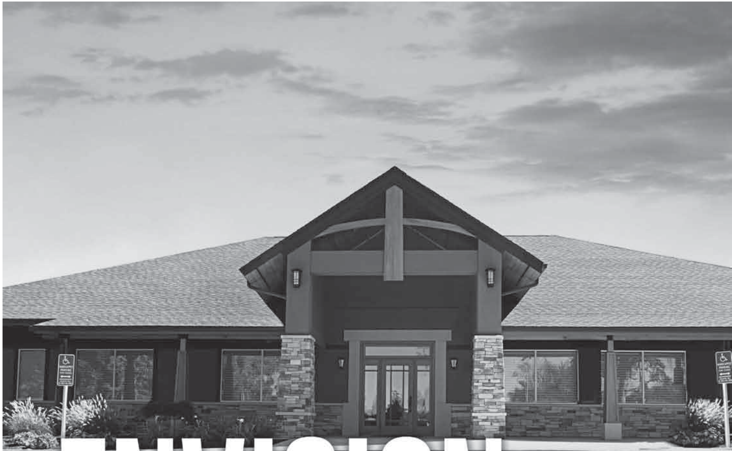
Recently-Completed Ground Up Construction Project
