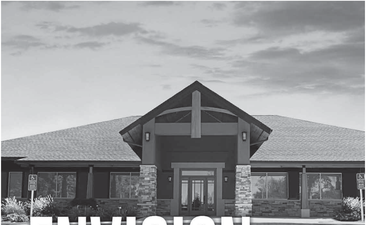
Recently-Completed Ground Up Construction Project
